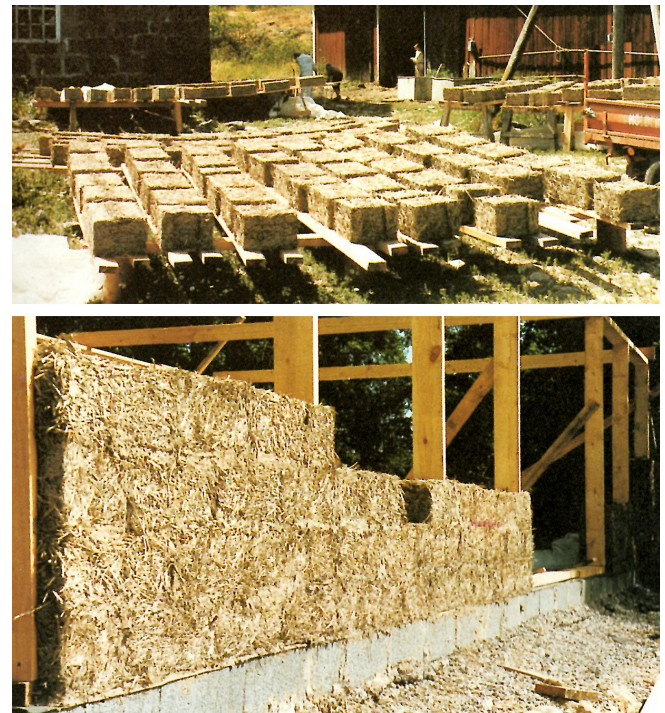
Figure 3. Mauritzberg Vacation House Prototype Construction. Sverre Fehn
