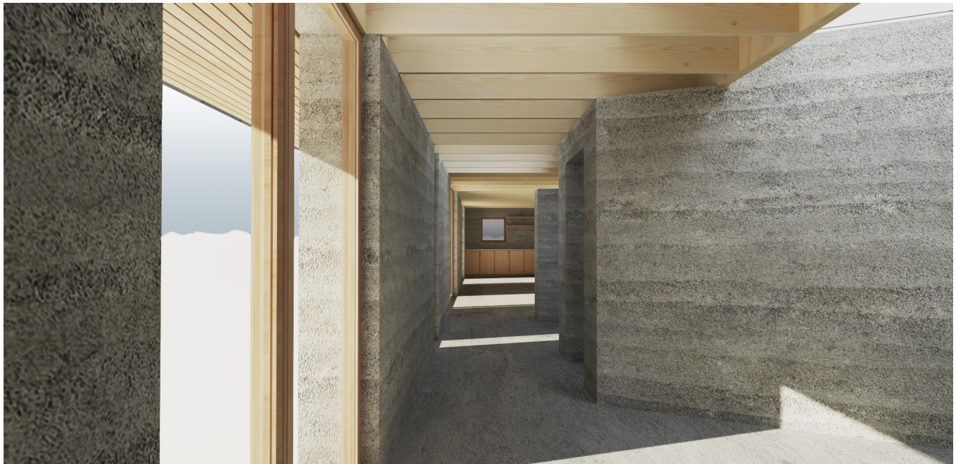
Figure 6. Hempcrete walls along interior passage
